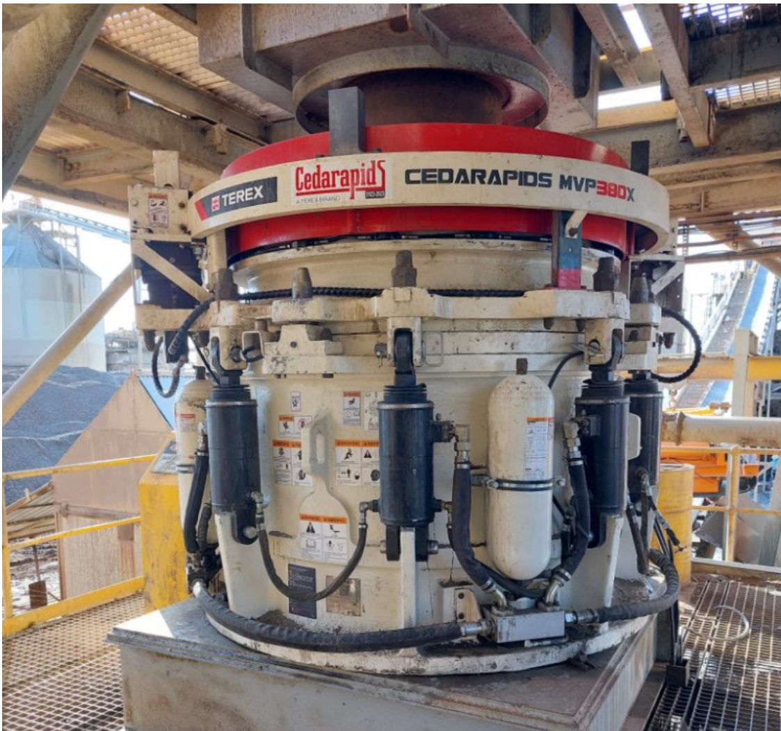
Figure 7 - New Terex 380 tertiary crusher installed
