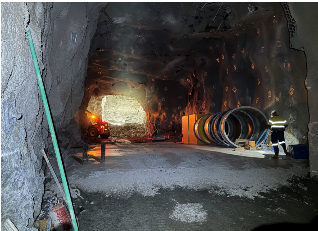
Figure 6 - Underground at Riverina showing the 4.5m diameter vent rise in the background and the cement pad poured as part of the primary fan installation (scheduled completion early December)
